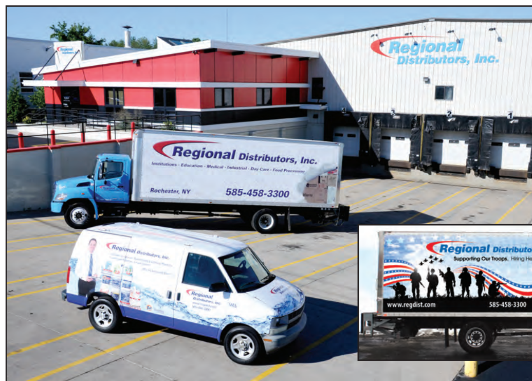
Regional Distributors’ state-of-the-art facility includes offices, a high-bay 60,000-square-foot warehouse and a large training room. The graphics on the truck shown in the inset indicate the company’s commitment to hiring U.S. military veterans.
